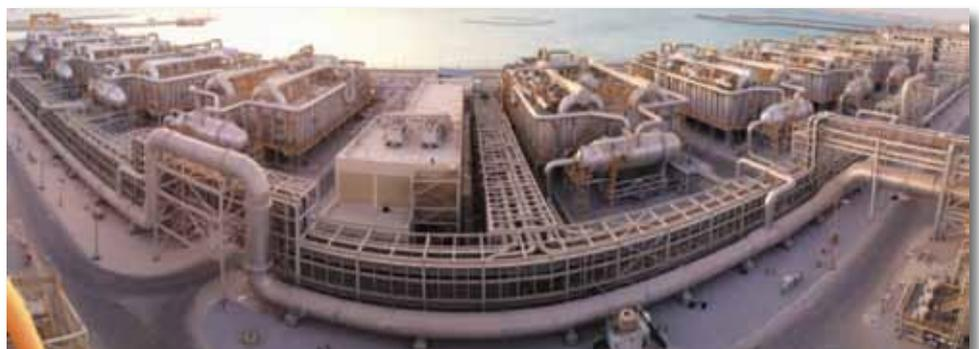
► Overview of MED Desalination (10 units) with interconnected water block piping rack
